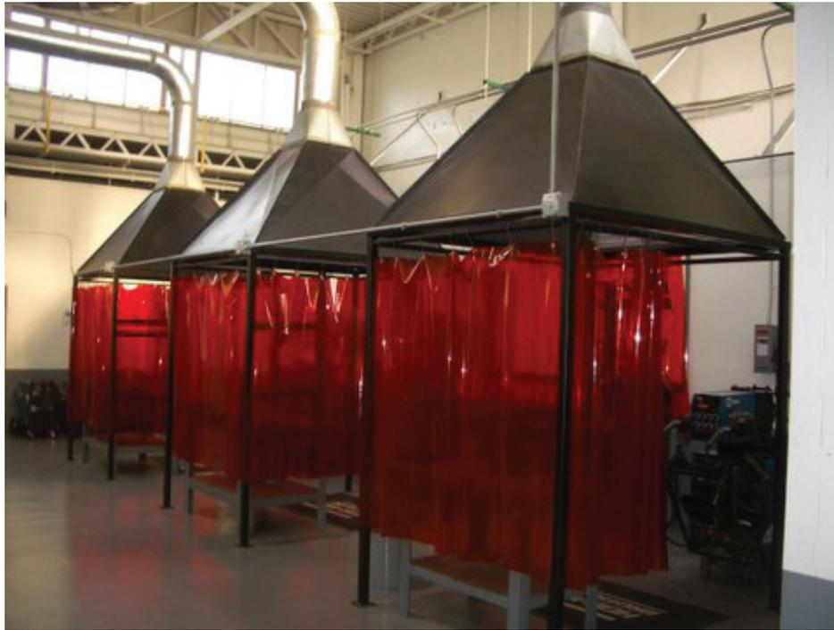
**Figure 14 - Welding booths with mechanical ventilation**
