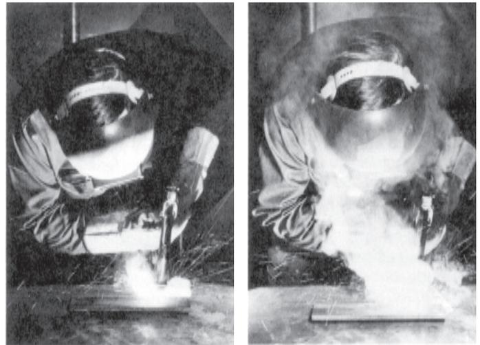
**Figure 17 - Smoke exhaust gun on and off.**
